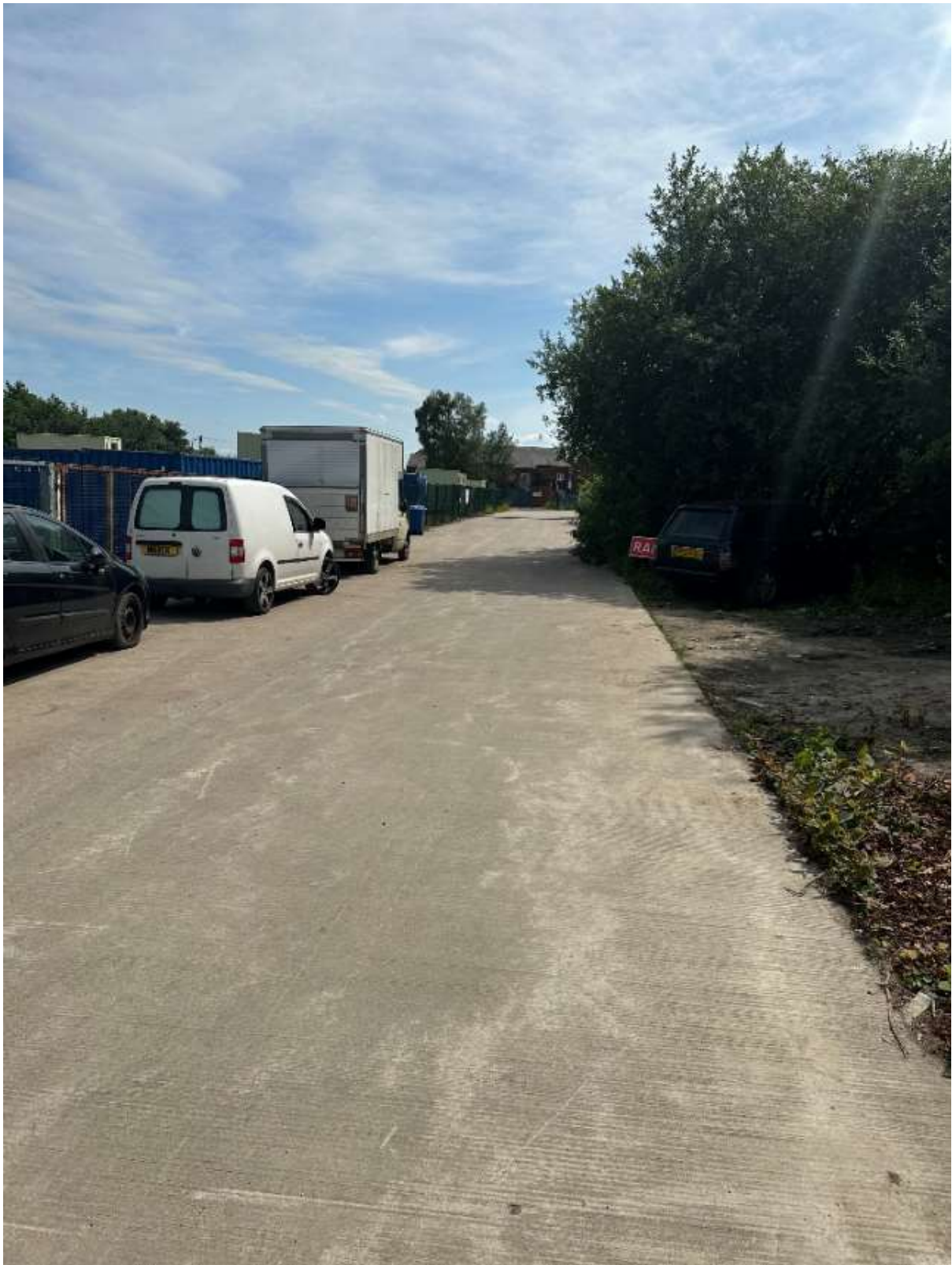
View of the private road.
